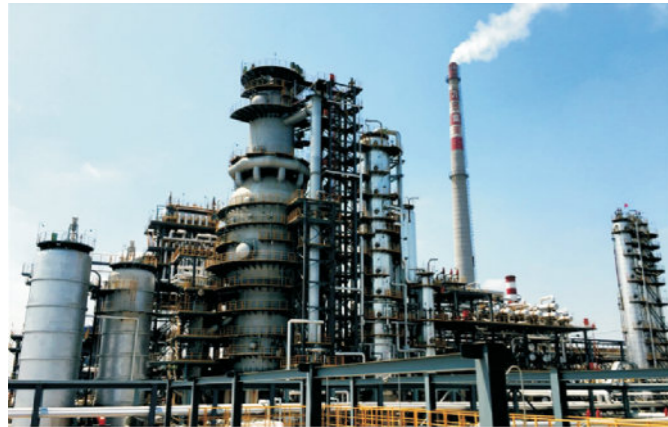
Dongying Liyuan Environmental Protection 1,800,000 tons/y DDC Combined Device
