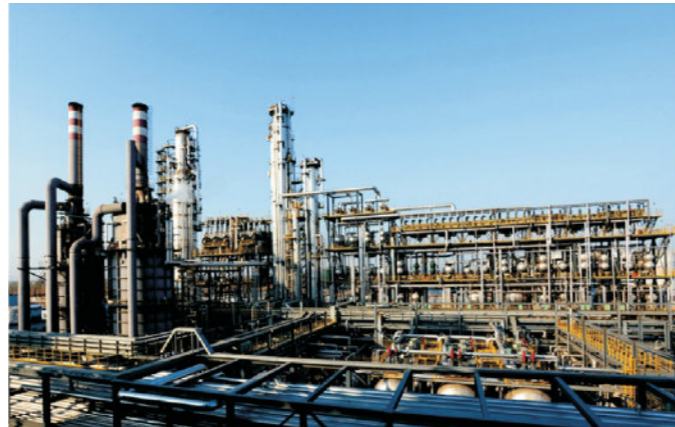
Shandong Wantong Petrochemical 6,500,000 tons/y Atmospheric & Vacuum Distillation Plant
